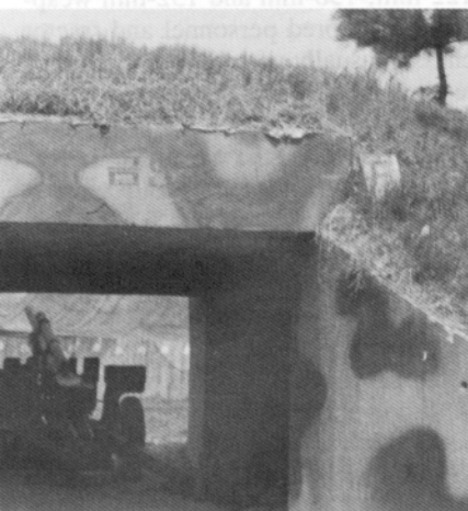
This ROKA 105-mm howitzer in a concrete bunker is aimed at the DMZ. Notice the thickness of the overhead cover.
