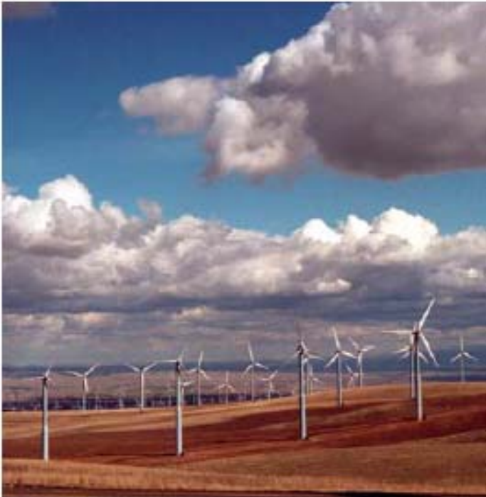
Stateline, Washington [399 x 660 kW = 263 MW]
