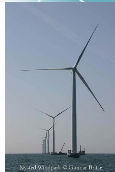
Nysted (Denmark) 72 x 2.2 MW = 158.4 MW [2003]
