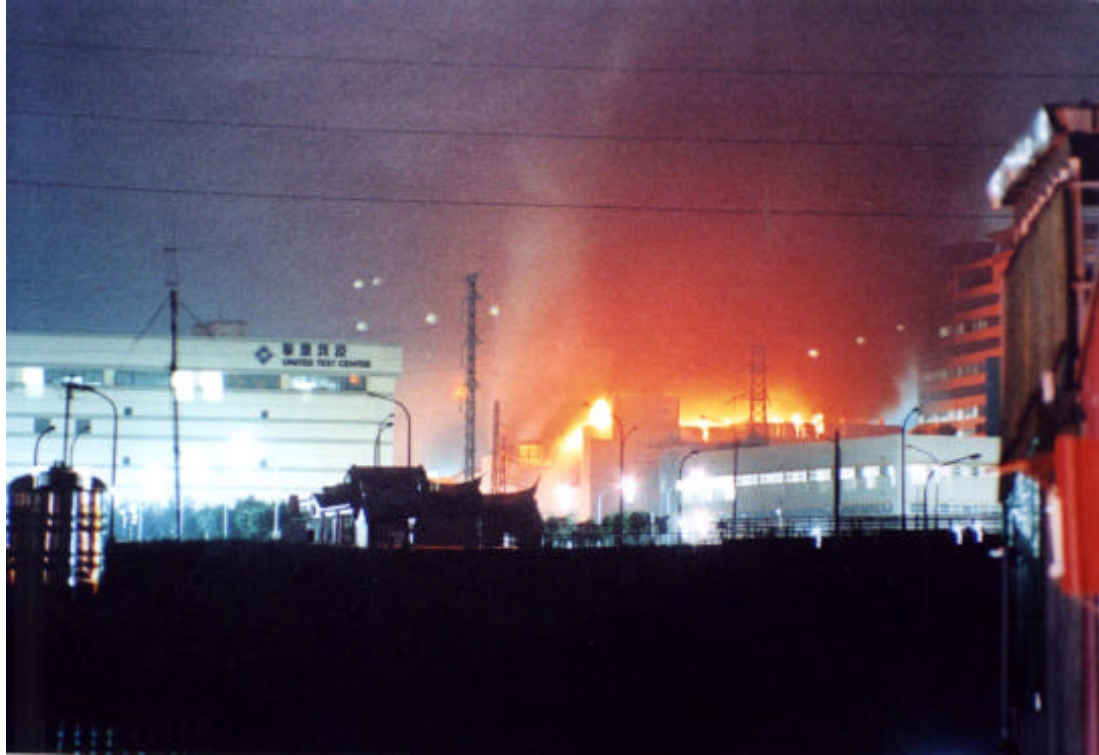
Fig. 2-1 The United Integrated Circuit's fire incident in 1997. Photo from Wu, Ching-ji.
